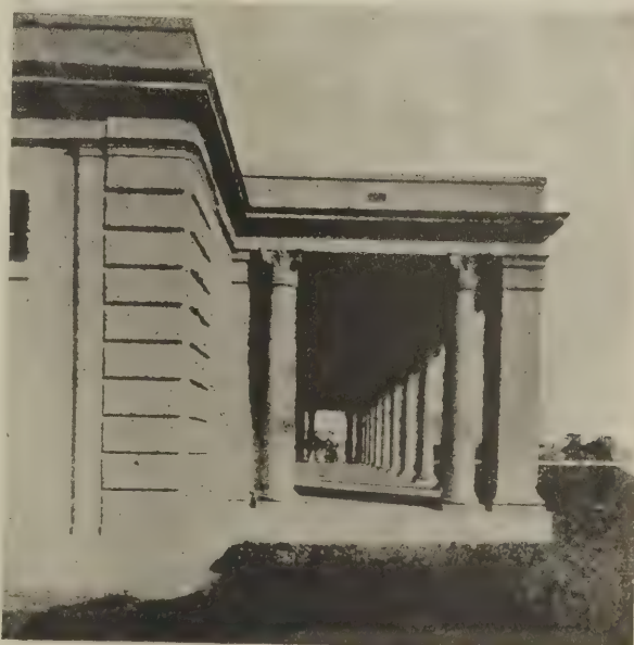
SOUTH PORTICO OF THE FIELD HOUSE, EAST POTOMAC PARK, WASHINGTON, D. C. THE PORTICO IS OF STUCCO ON TERRA COTTA TILE. BOTH CONCRETE AND STUCCO ARE OF THE EXPOSED AGGREGATE TYPE AND ARE OF THE SAME COLOR AND TEXTURE
